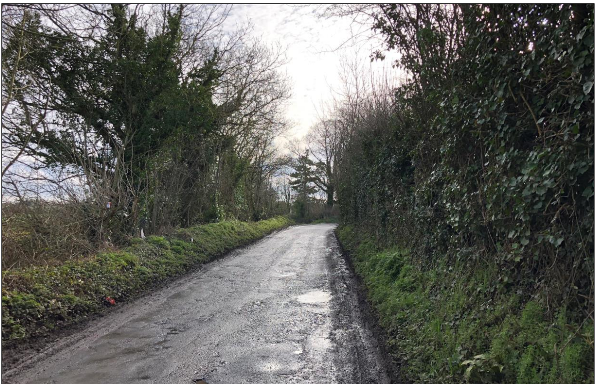
Figure 5.0 The Rathmullan Road runs alongside the northern, eastern and southern boundaries of the subject site.
